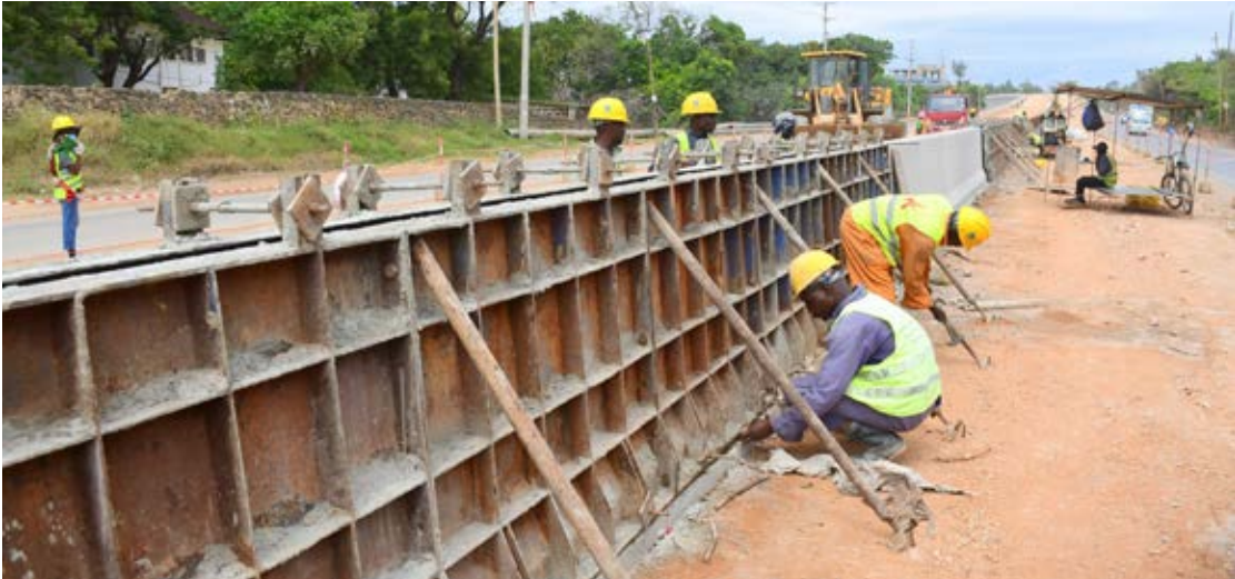
Nyali Bridge–Mtwapa Bridge section under construction in Mombasa.
